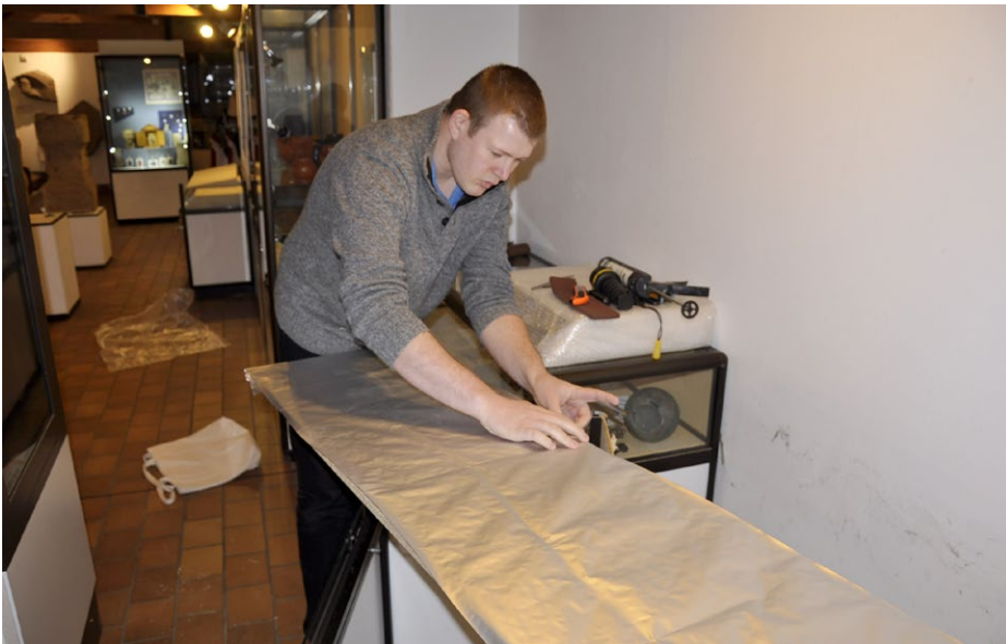
Fig 28. Wrapping a wood board with Marvelseal 360 and 3M 425 tape to stop emission of harmful gases from the wood into a showcase
