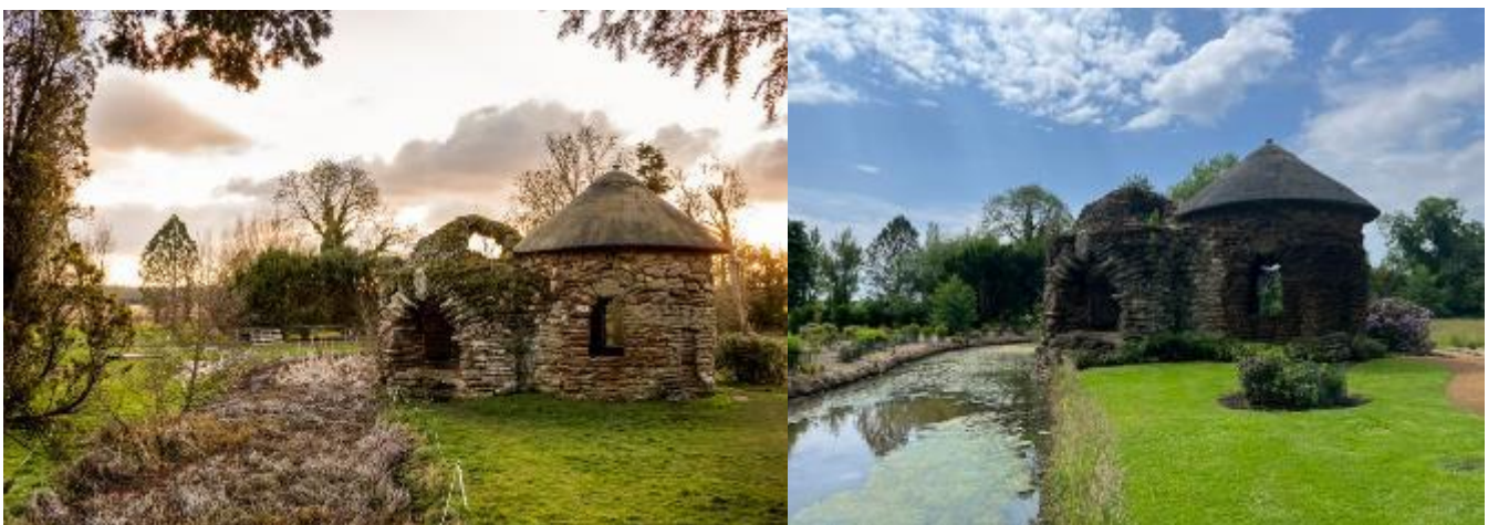
Figure 6 (before) and Figure 7 (after) - Key to the restoring the garden throughout Wrest Park was an understanding of the site's hydrology. Waterlogging had undermined the establishment of new planting in previous attempts to rejuvenate the 18th century gardens. Here we see the Bath House Water, before and after dredging and re-presentation.
